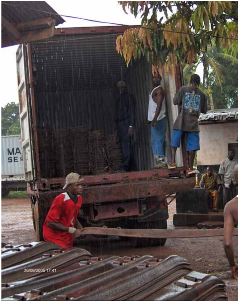
Unloading sleepers at Port Loko Police Station. – 26 Sept. 2005. Wood was used to cover and hide the sleepers.
